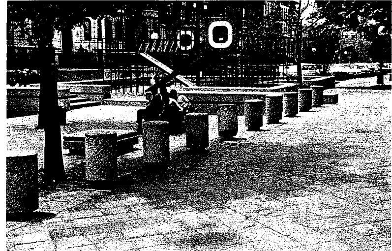
FIG. 41. Pedestrian Area, St. Marks Avenue. View of play equipment and parking area. The rear portion of the street is not open to through-traffic. The only visible sign of vandalism is the broken concrete piling which was hit by a city sanitation truck. (Photo by author)
