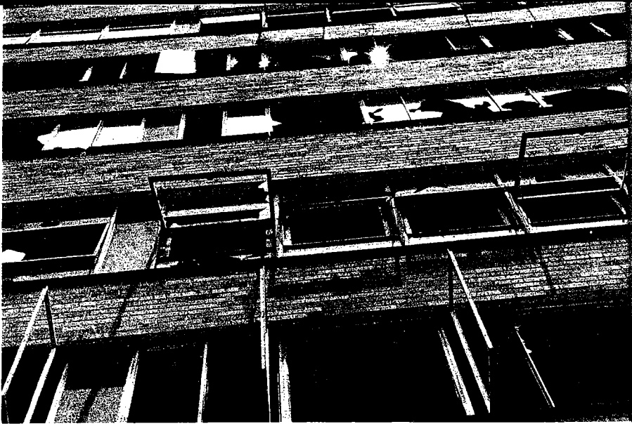
FIG. 6. Pruitt-Igoe, St. Louis, Missouri. View of vandalism to windows of public access galleries serving upper levels of the buildings. (Photo by Bob Williams)
