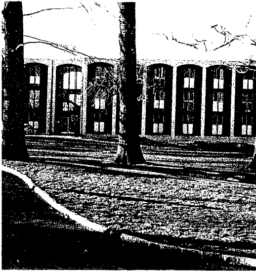
FIG. 56. New Dormitories, Sarah Lawrence College. The new dorms are tied together in one long double-loaded slab structure, not unlike a motel. Students in the new dorms feel isolated without any sense of community. It is claimed by college counselors that the students easily fall into patterns of antisocial behavior. (Photo by author)
