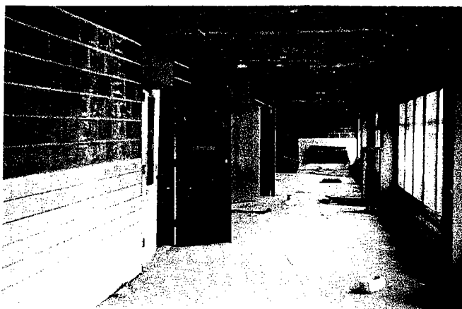
FIG. 38. Actual View of Pruitt-Igoe Gallery Area. View of what was intended by the architects to be highly-used public gallery (see fig. 37). These corridors are not juxtaposed with apartment units and so are feared by residents and unused. The open doors lead to what were once laundry rooms. (Photo by author)
