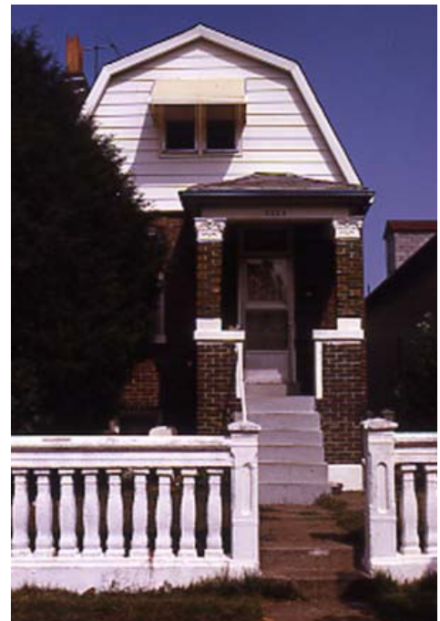
Fig. 26. Poured concrete fence 2
