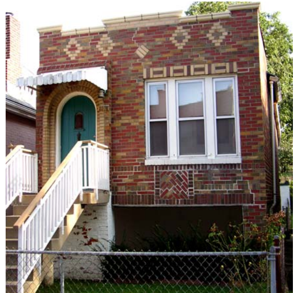
Fig. 21. Patterned brick façade
