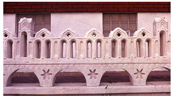
Fig. 25. Poured concrete fence 1
